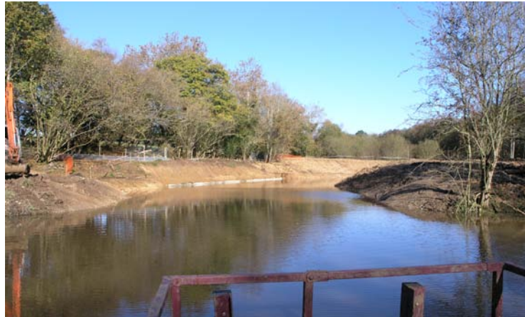
Looking NE from the entrance to Timsbury canal.
